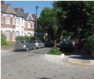
Raised junction, Haringey
